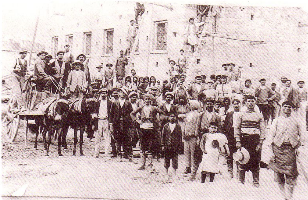
MALE AND FEMALE WORKERS, ENGAGED IN BUILDING THE BERENGARIA HOTEL AT PRODROMOS IN 1928.
